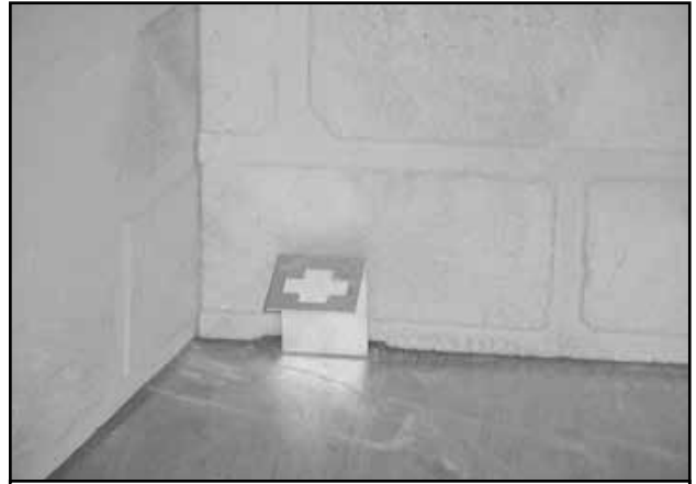
Figure 8.8 Grate Retaining Bracket in Place
