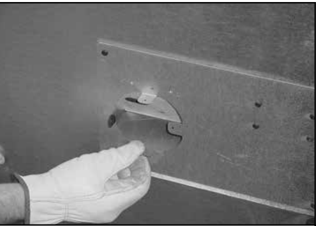
Figure 3.19 Bending Tabs on Outside Air Kit Collar
