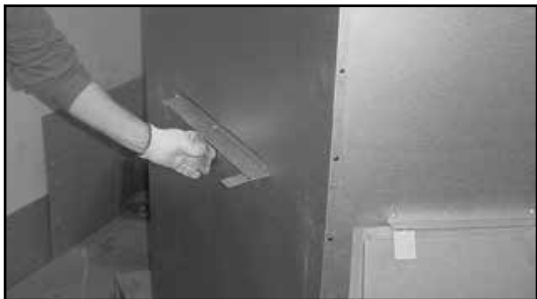
Figure 3.7 Bend Refractory Brackets Back Down
