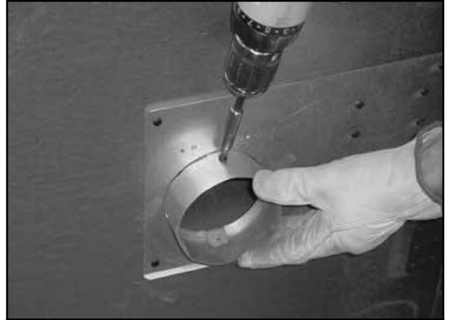
Figure 3.20 Attaching Outside Air Kit Collar
