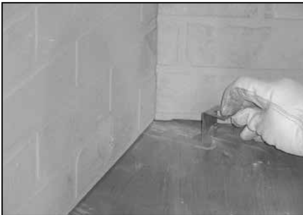
Figure 8.7 Slide Grate Retaining Bracket into Notch
