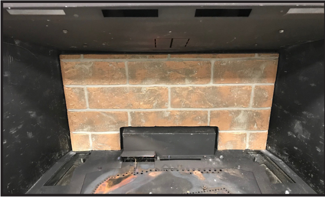
Figure 4 Back Refractory Installed
