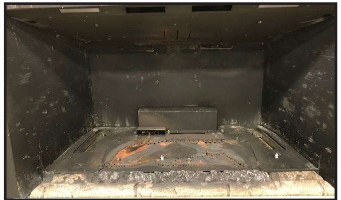
Figure 3 Base Refractory Installed
