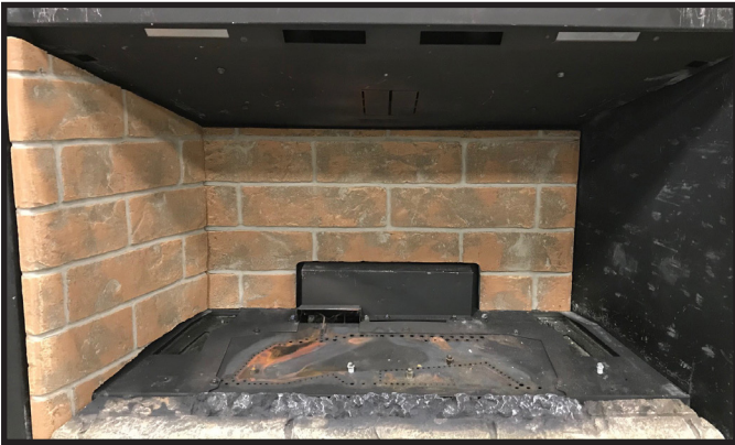
Figure 5 Left Refractory Installed
