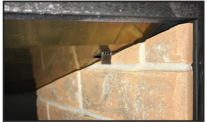
Figure 7 Right Refractory Handbend Tab
